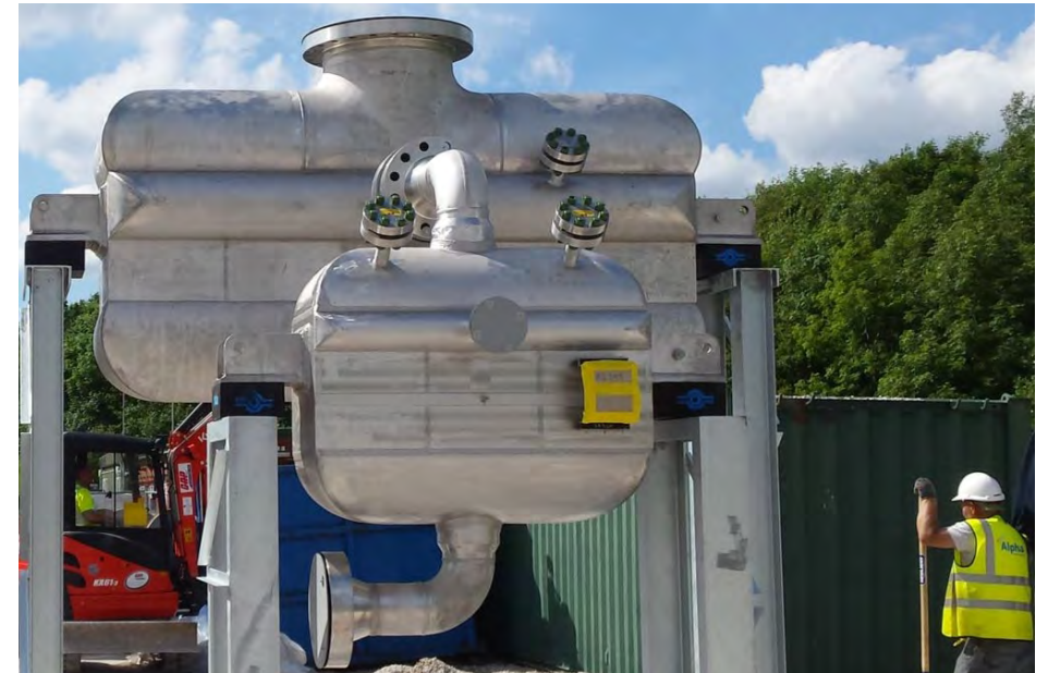
Bury Demo site Evaporator and HX1 (front)
