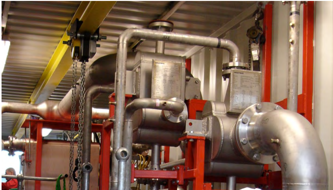
Slough test site PCHes
